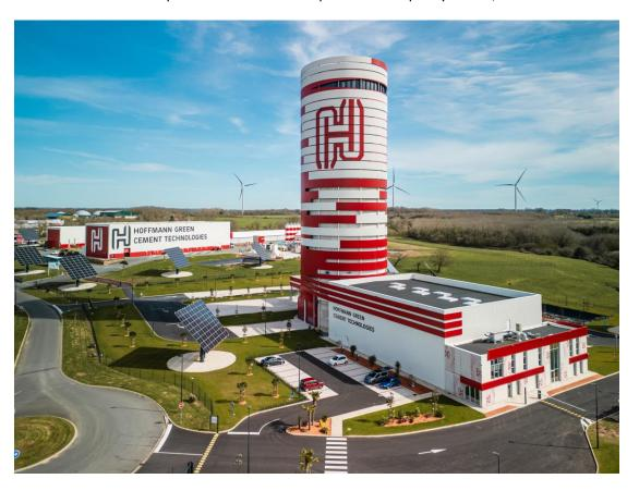
The "H2" production unit, which is 70 metres high, is based on a "gravity" process and built entirely of Hoffmann Green concrete. It has production capacity of 400,000 metric tons of cement per year operating 3x8 shifts. This unit model is the one that will be duplicated for the Company's developments in France and internationally.
